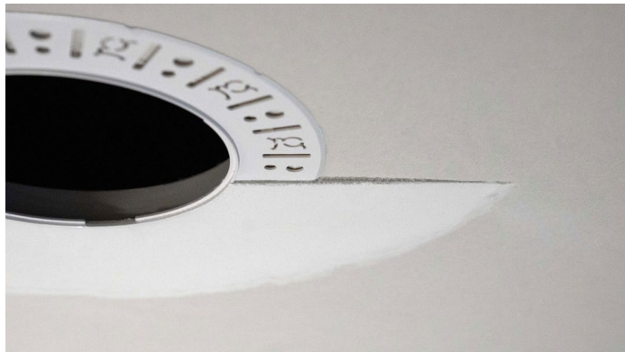
Partially finished mud ring, showing cross-section detail.
