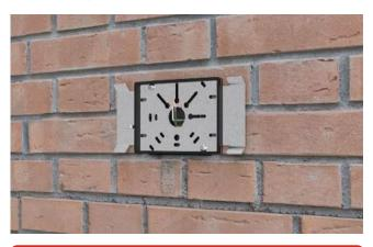
1. Install the luminaire mounting bracket.
