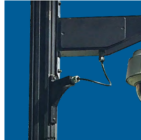
Auxiliary Channel Exit
