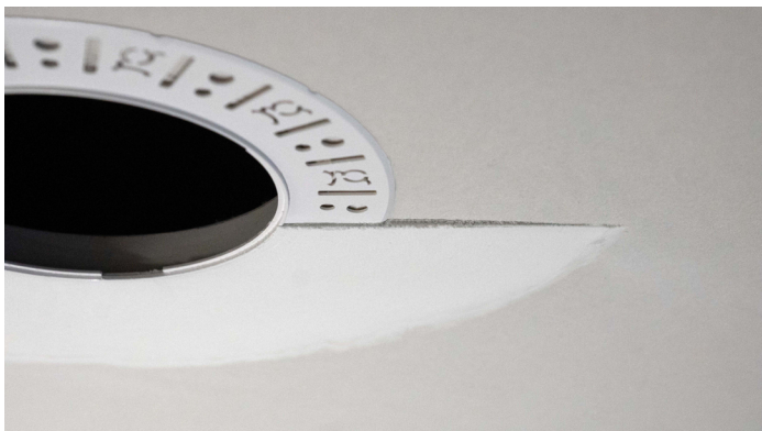
Partially finished mud ring, showing cross-section detail.
