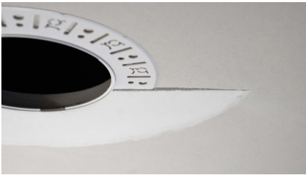
Partially finished mud ring, showing cross-section detail.
