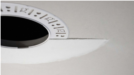
Partially finished mud ring, showing cross-section detail.
