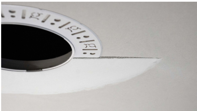
Partially finished mud ring, showing cross-section detail.
