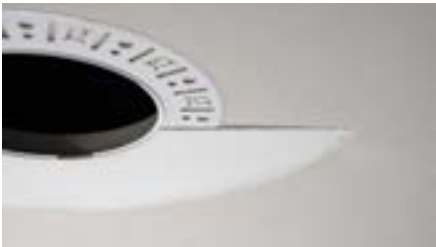
Partially finished mud ring, showing cross-section detail.
