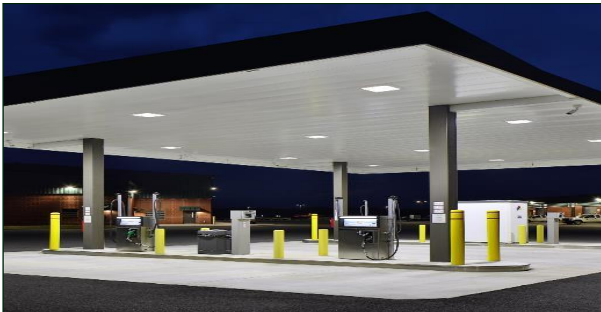
P CNY Petroleum Canopy
