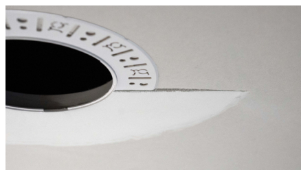
Partially finished mud ring, showing cross-section detail.
