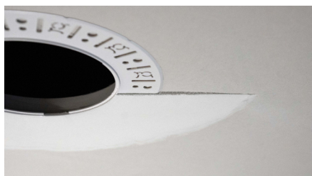
Partially finished mud ring, showing cross-section detail.
