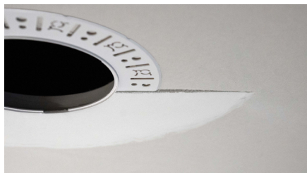
Partially finished mud ring, showing cross-section detail.
