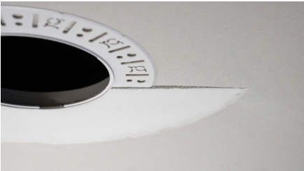
Partially finished mud ring, showing cross-section detail.
