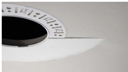
Partially finished mud ring, showing cross-section detail.
