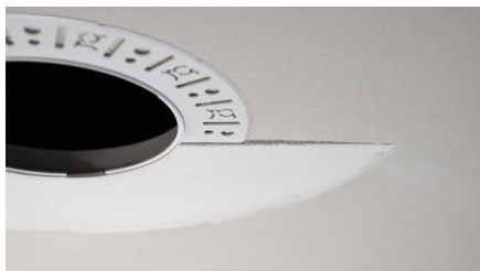
Partially finished mud ring, showing cross-section detail.
