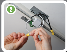
Connect track to mounting plate and wire.
