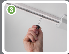
Attach track to ceiling.
