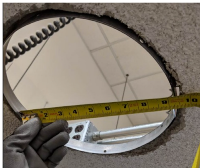
Measure the diameter of the metal frame through the center of the opening
