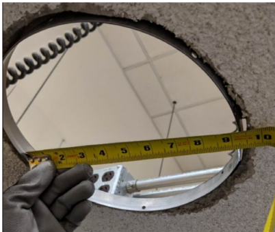
Measure the diameter of the metal frame through the center of the opening
